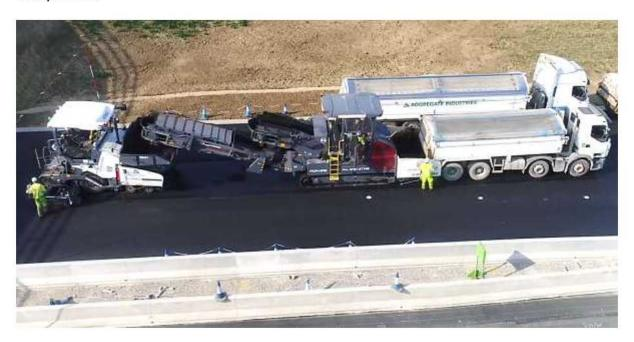
Section 3: The final layer of road surface is now being laid (see picture above) and white lines and other road marking will begin in the next few weeks. The last bridge over the A14 Huntingdon southern bypass, at New Barns Lane, is now structurally complete, with kerbing underway ahead of surfacing.
